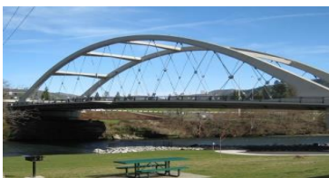
Depot Street Bridge at John F. Fleming Memorial Park
